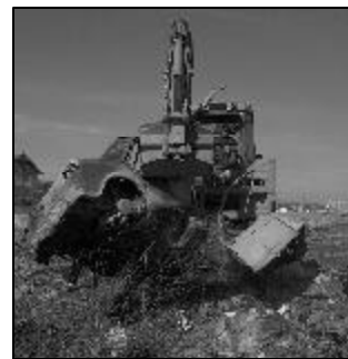
A Kosovo Protection Corps engineer pulls an abandoned car out of a ditch near the culvert on Ring Road.
